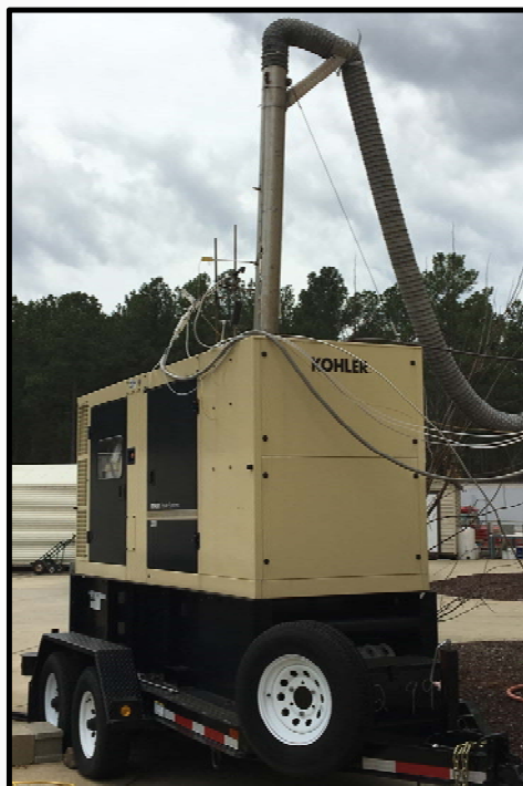
AEMD's Stationary Diesel Facility (200kW genset)
